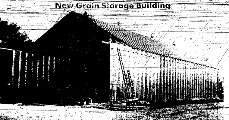
ERECTOR OF A NEW 150,000-BUSHEL grain storage building for Wayne Grain and Feed co., Wayne, was completed Wednesday. The new structure, located between Logan and Nebraska streets on East Second, will be used to store corn under CCC loan. The structure is 150 feet long and 50 feet wide.
